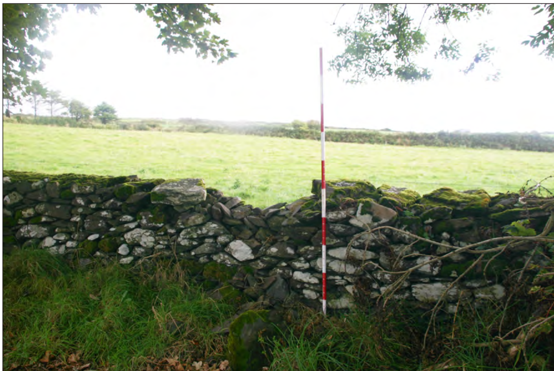
Plate 12: Detail view of damaged and partially breached section of eastern boundary wall
