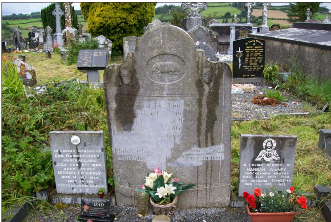
Plate 11: View of damage caused by recent attempts at cleaning the headstone
