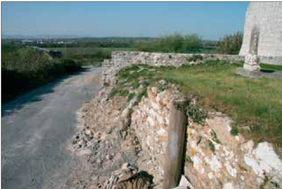
Plate 13: View from south of collapsed breach in north-west corner of west boundary wall
