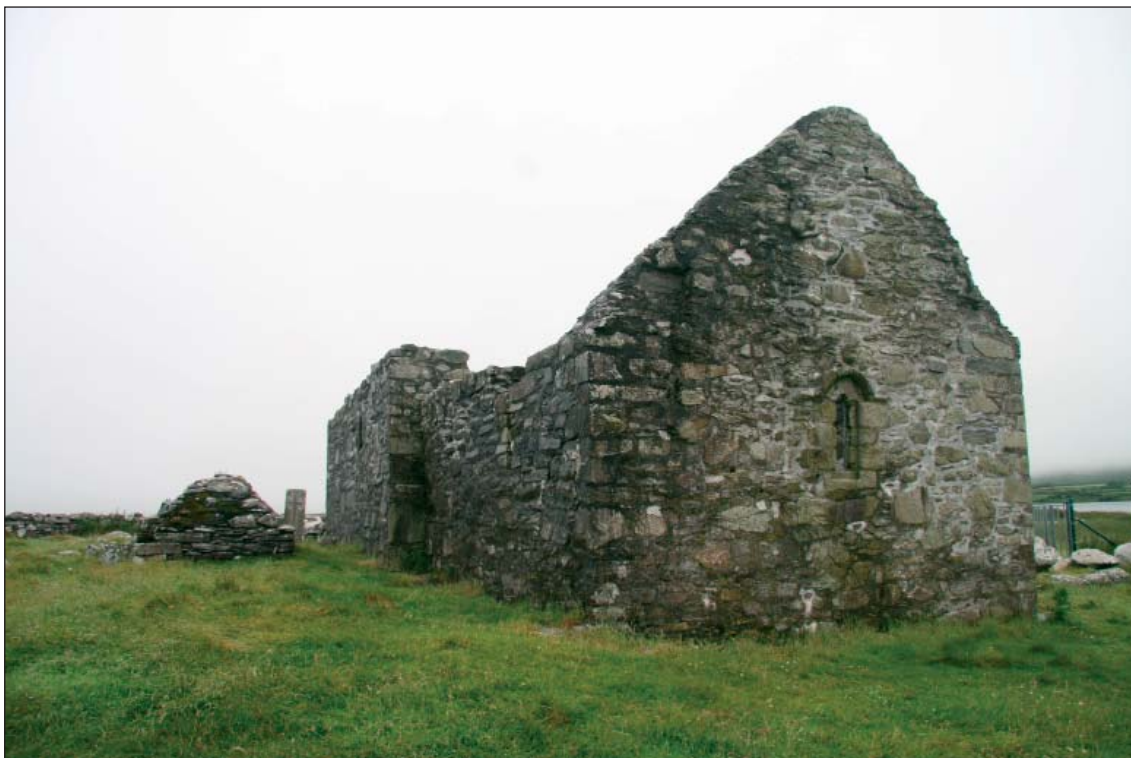
Plate 1: View from S-E of interior of Church Island burial ground. Note the absence of the E gable buttresses and the two abutting tombs at the S elevation
