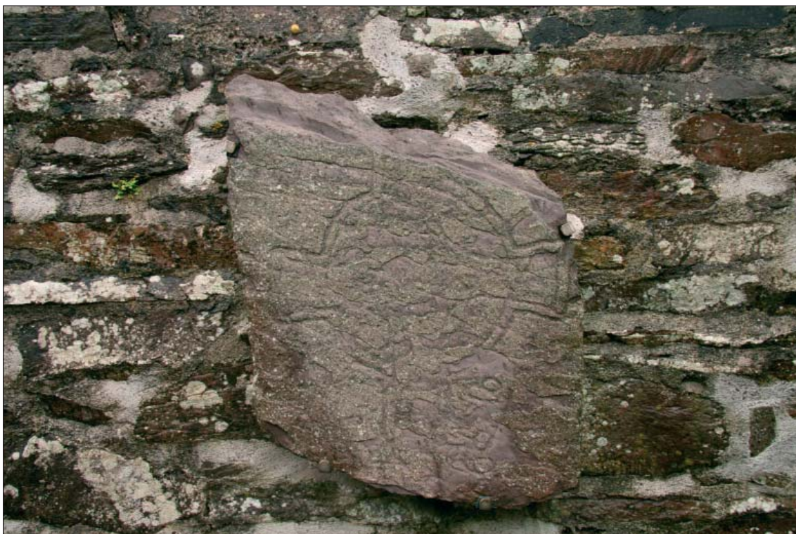
Plate 15: Close-up view of cross-slab CS7 on the nave of the church. Note the fresh spalling at the top and the surviving patch outer lamination of its face
