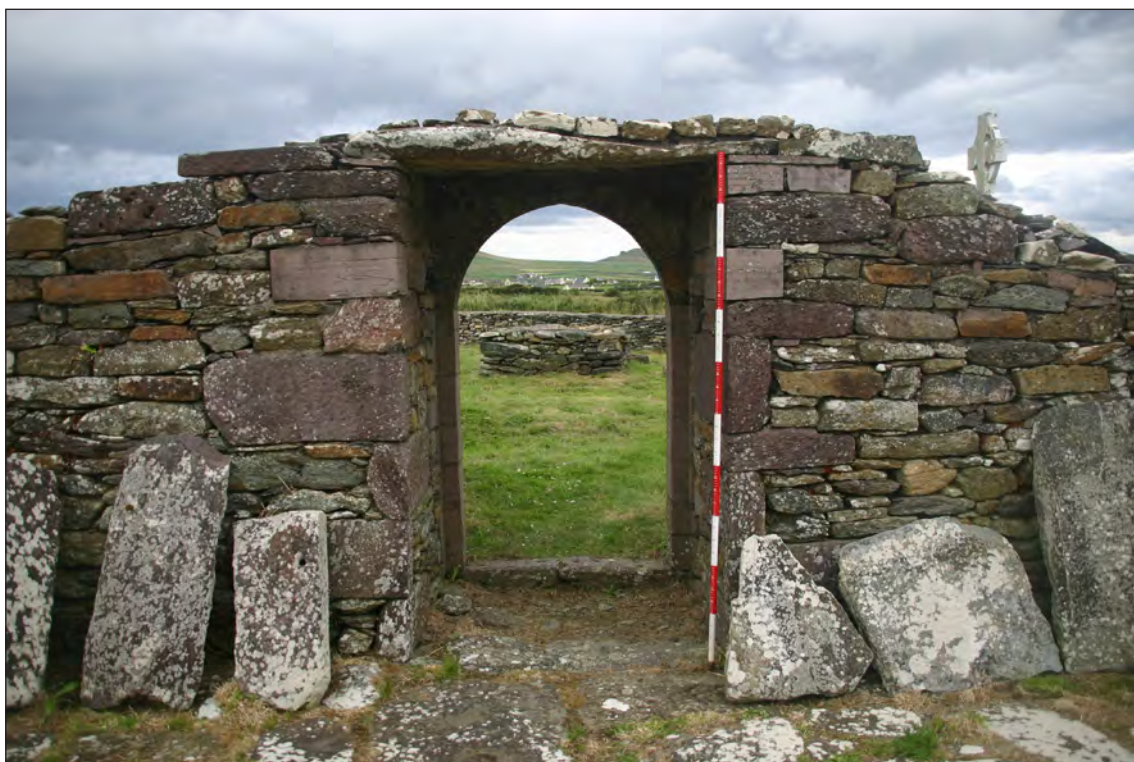
Plate 12: View of interior of N doorway of Dunurlin Church. Note extent of rebuilding works undertaken in 1991. Further note medieval architectural fragments lying loose against wall
