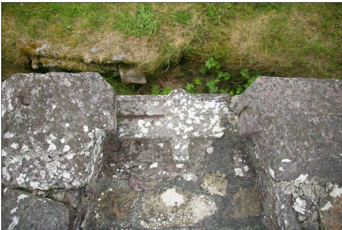
Plate 17: Overview of basal limits of chamfered, splayed embrasure of E window. Note projecting 'V' base for centre mullion to accommodate twin lights. Further note glazing slots to base and side stones. Note also pivot stone for window shutter
