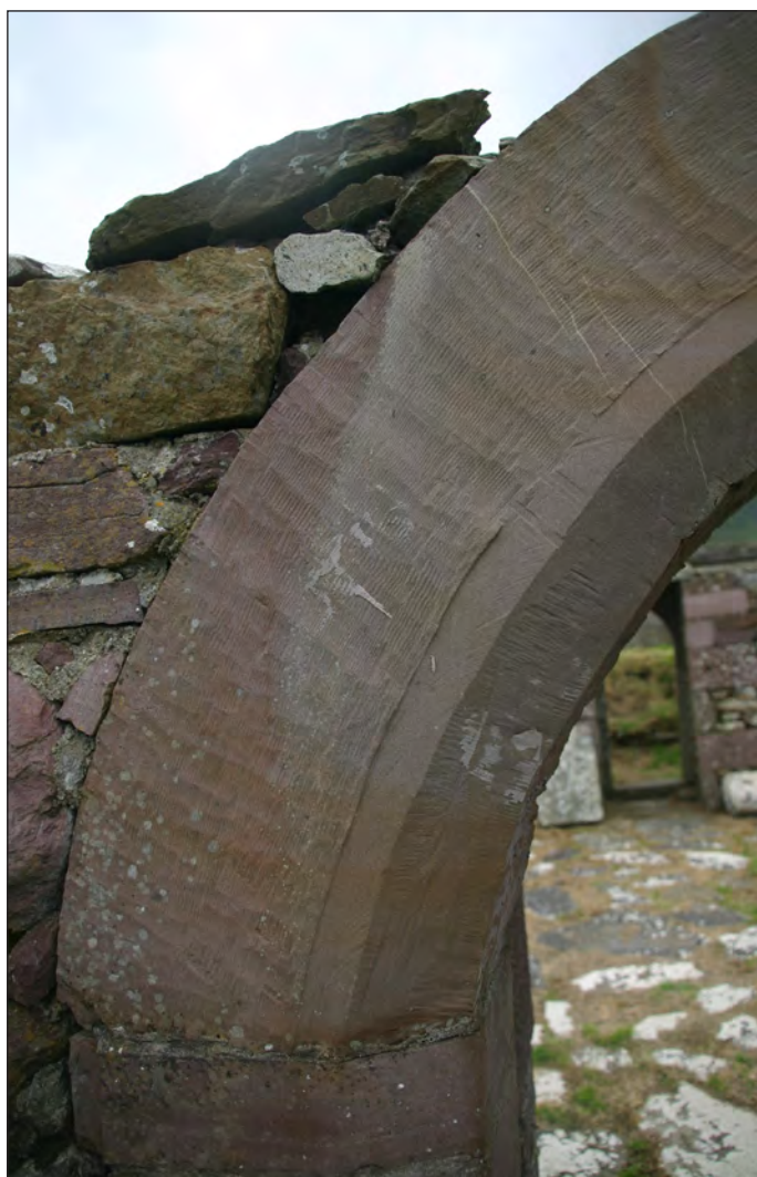
Plate 14: Close up view of very poor work on replacement arch stone on N doorway of Dunurlin Church. Note extensive amateurish, inappropriate machine and angle grinder marks
