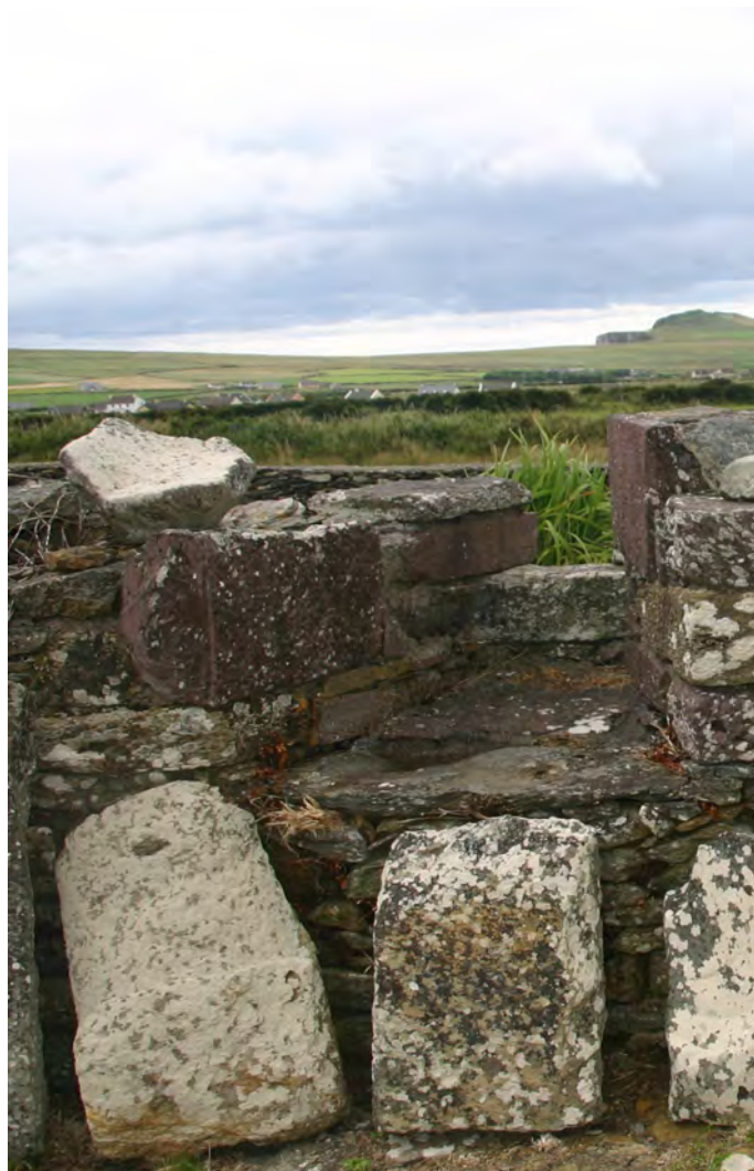
Plate 19: Interior view of splayed embrasure of N window in Dunurlin Church. Note architectural fragments against wall and broken font fragment lying loose on top
