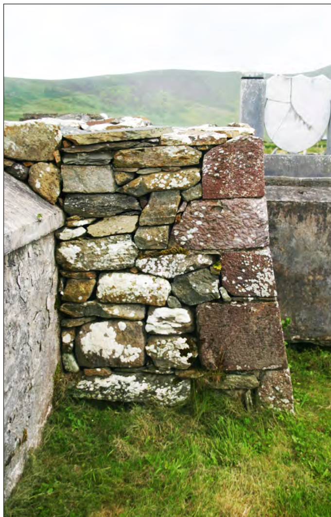
Plate 15: View NW corner of Dunurlin Church. Note sharp basal batter and well dressed, matched quoins
