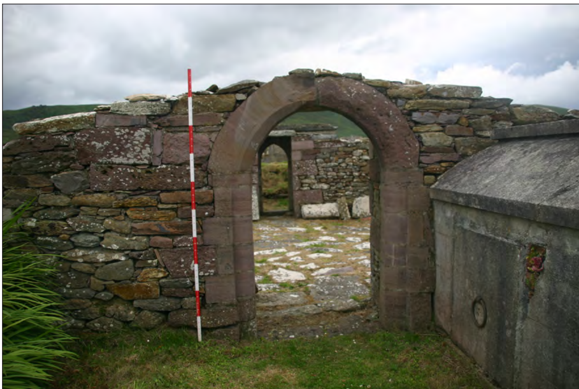
Plate 13: View of exterior of N doorway of Dunurlin Church. Note extent of rebuilding works undertaken in 1991
