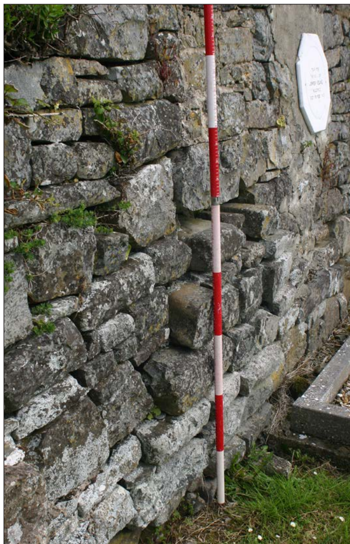
Plate 11: View of noticeable outward bulge directly beneath easternmost window on southern elevation
