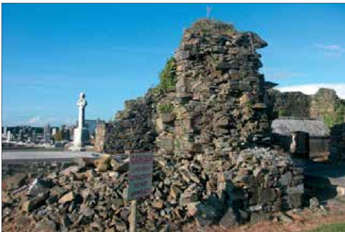
Plate 5: View of collapsing south-west section of south elevation of Kilfeighney church
