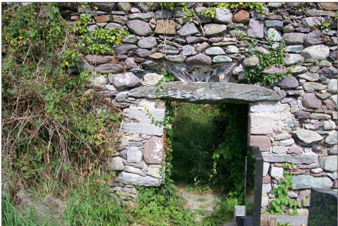
Plate 8: Exterior view of flat-lintelled doorway in southern elevation, taken from south
