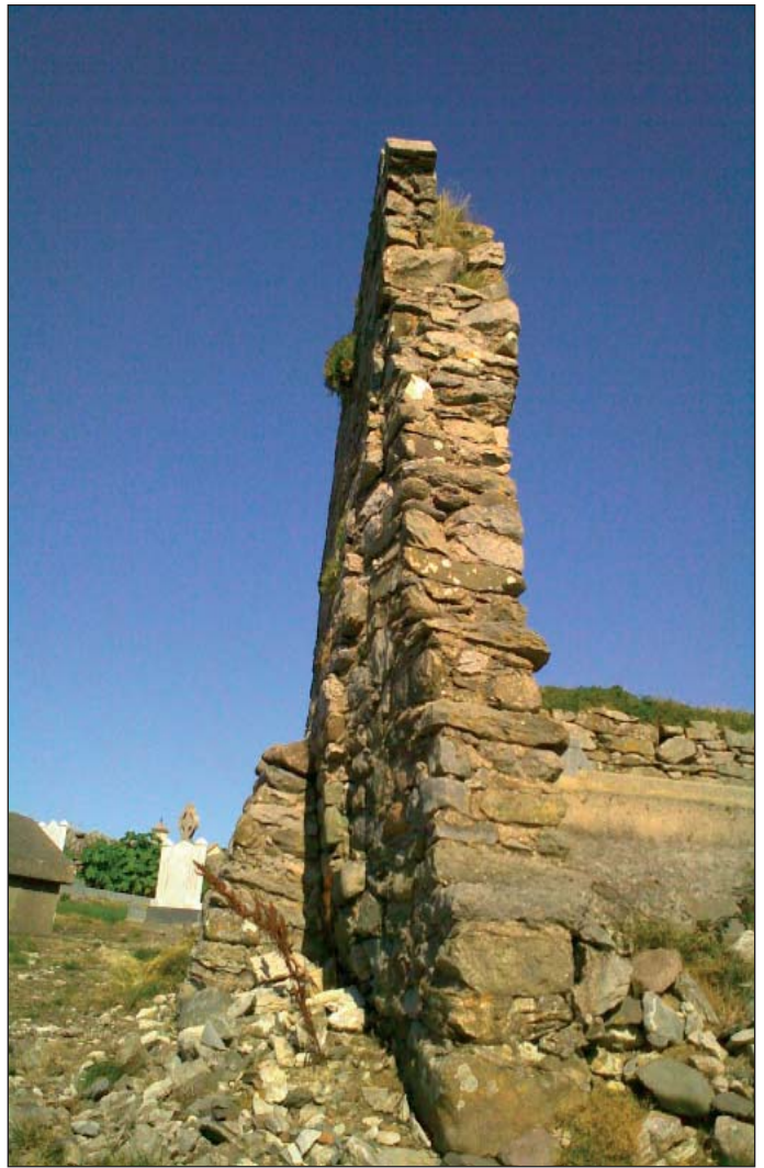
Plate 3: Side view image by the author from the exterior SW corner of extant W gable in 2009. Note inadequate low buttress and outward or westerly bulge
