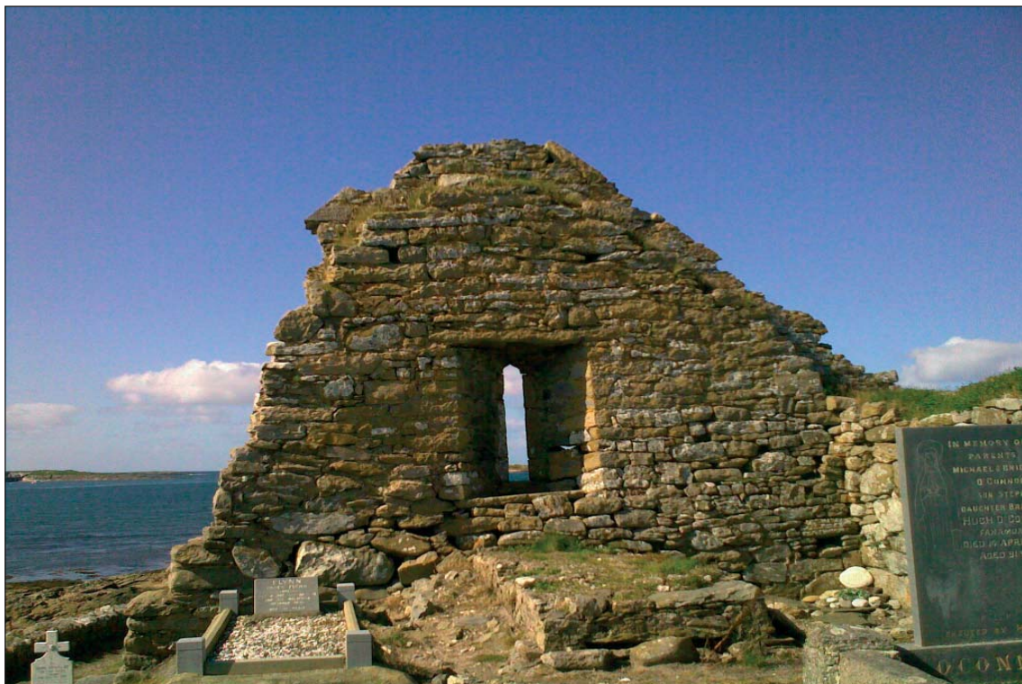
Plate 2: View from E of W gable of Kilshannig church. Image taken by author in 2009. The W gable collapsed in January 2011. Note coherent leaning and fracturing on the S side and S basal area of the W gable. Further note low rectangular tomb and Flynn burial plot
