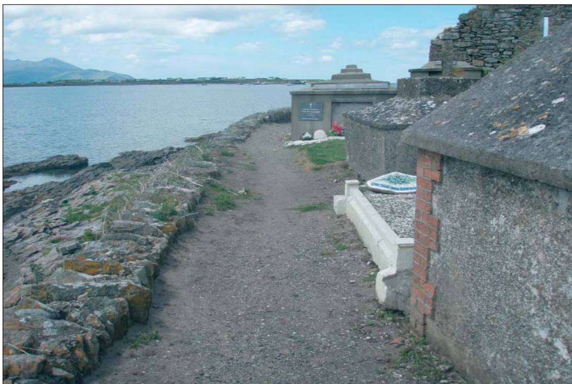
Plate 14: View of curving S section of interior gravelled pathway and very low section of boundary wall. Note only 'soldier' capping of wall visible here
