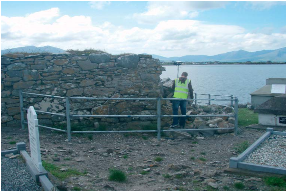
Plate 6: View of collapsed NW corner of N elevation of Kilshannig church from N. Note robust railing around it erected by KCC
