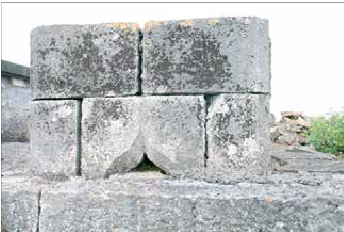
Plate 18: Close up view of upper tier on Corridan Tomb 44. Note all masonry in image constructed with medieval church masonry including 15th century ogee head of single light
