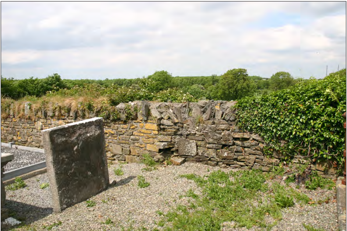
Plate 4: View of northern section of boundary wall. Note poor repair and ivy growth
