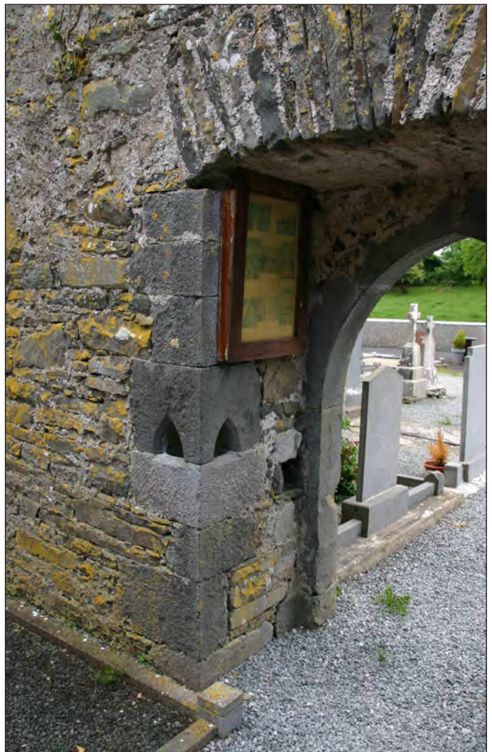
Plate 21: View of inner eastern side of doorway on south elevation. Note double-entry stoup, similar to Carrigafoyle and Aghavallen churches
