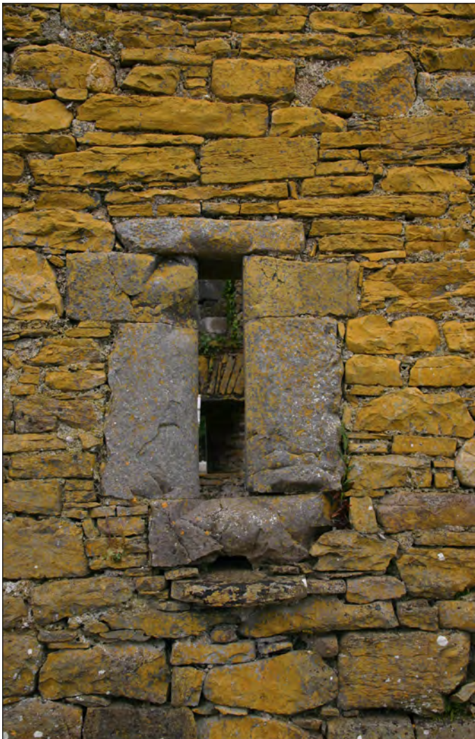
Plate 20: View of small narrow flat lintelled window. Note water outlet beneath cill
