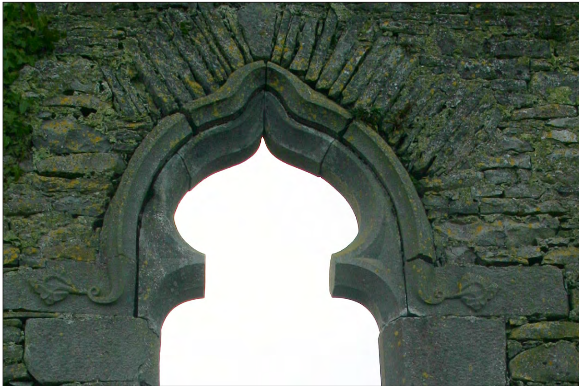
Plate 24: Close up exterior view of ogee head of east window. Note vine-leaf motifs to terminals of hood moulding. Further note missing centre mullion
