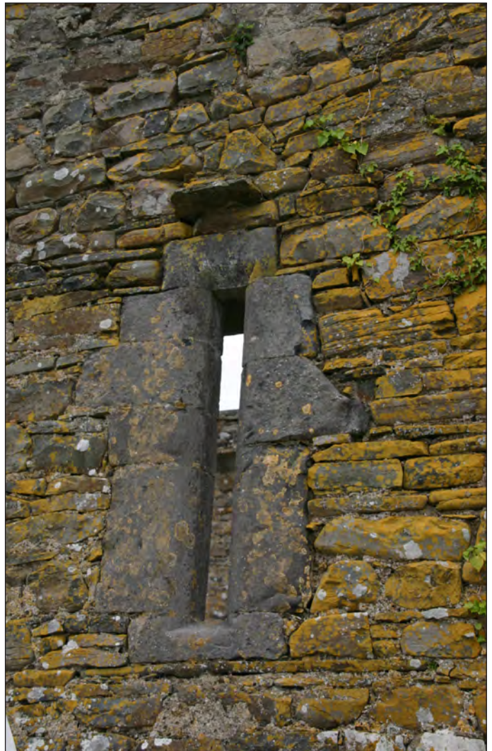
Plate 19: View of flat lintelled narrow window. Note projecting drip flag over it.
