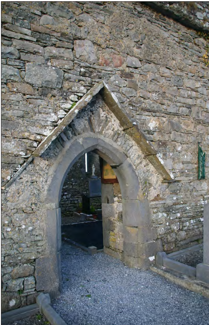
Plate 18: View of entrance doorway on south elevation. Note featured canopy or hood over
