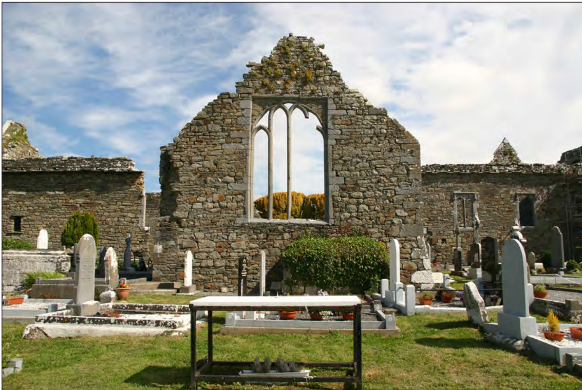
Plate 8: Exterior view of south gable of south transept. Note lancet type lights set within rectangular surround. Further note simple outdoor altar
