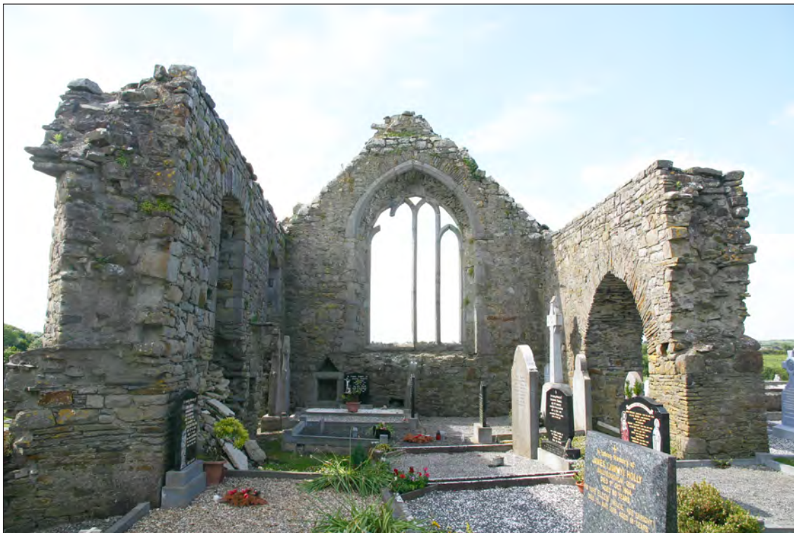
Plate 9: View of interior of south transept. Note inappropriate modern masonry splay to north-east ragged terminal of transept (bottom left of plate). Further note the extent of the burials and the central depression of the ground
