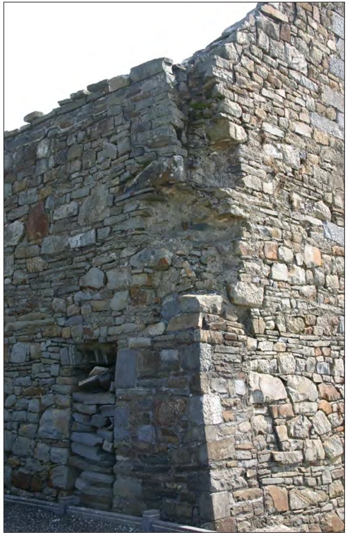
Plate 13: Exterior view of collapsed south-west angle and corner buttress of south-transept
