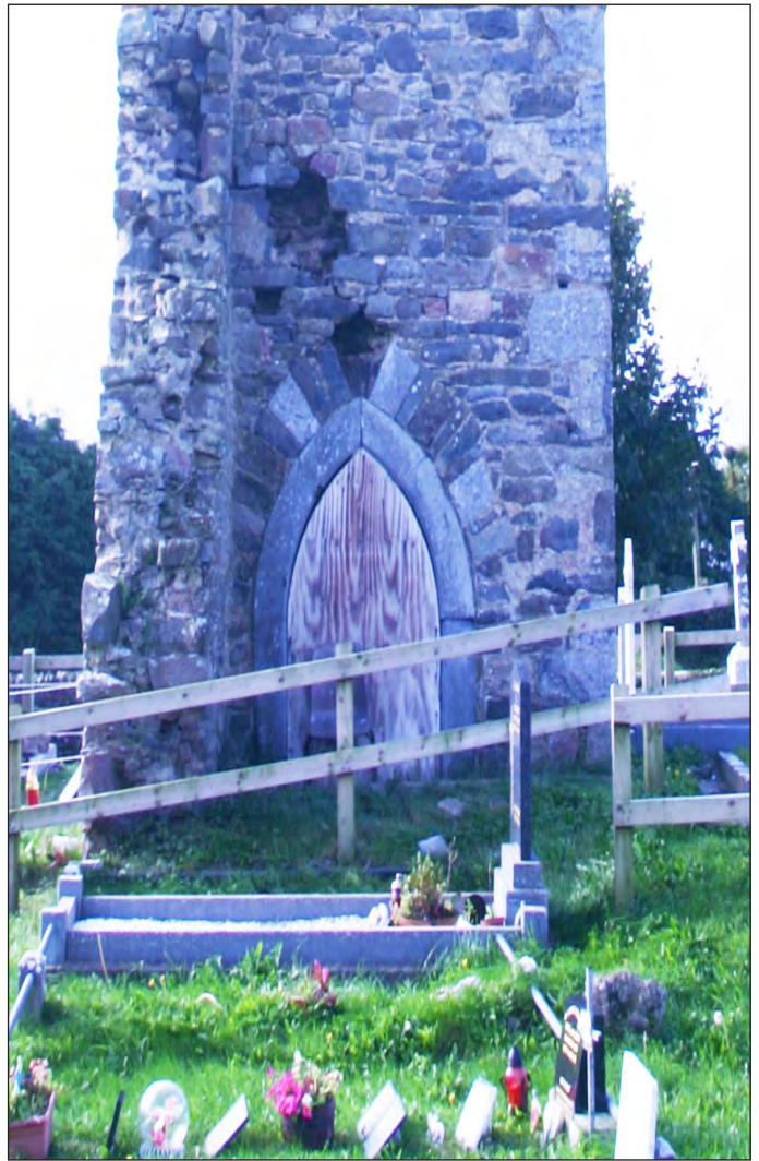
Plate 25: View of boarded up entrance to tower on north elevation. Note missing keystone and other masonry voiding
