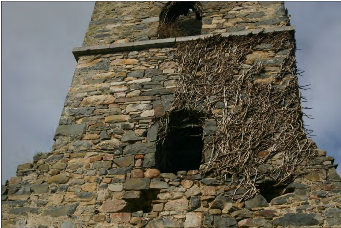
Plate 27: View of 1st floor level of east elevation. Note remains of recently removed vegetation, poor nature of masonry joints and voidings
