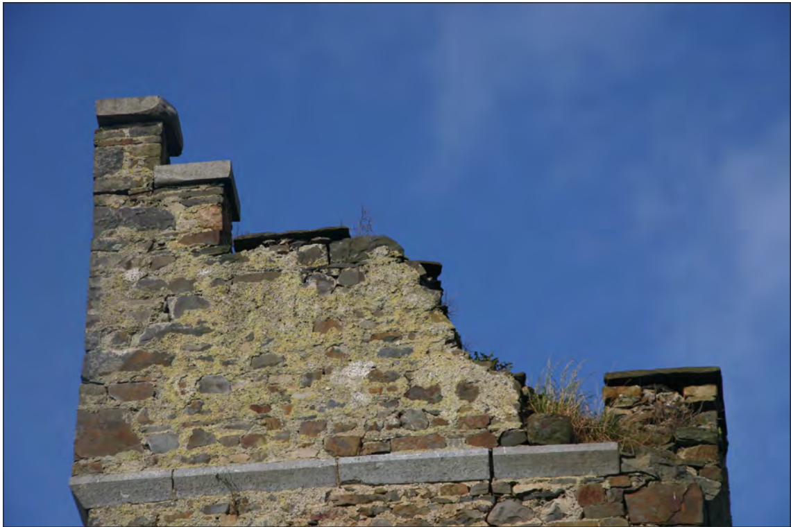
Plate 23: View of damaged crenellations on parapet on east elevation of tower
