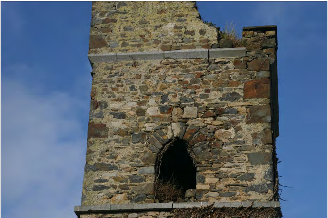
Plate 24: Close up view of 2nd floor and upper limits of east elevation. Note coherent crack in masonry extending to window opening from parapet collapse area
