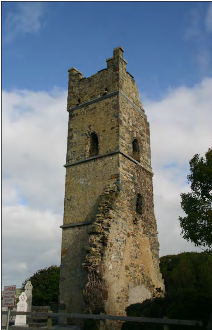
Plate 22: View of south-east angle of tower. Note ragged remains of nave of church acting like buttress
