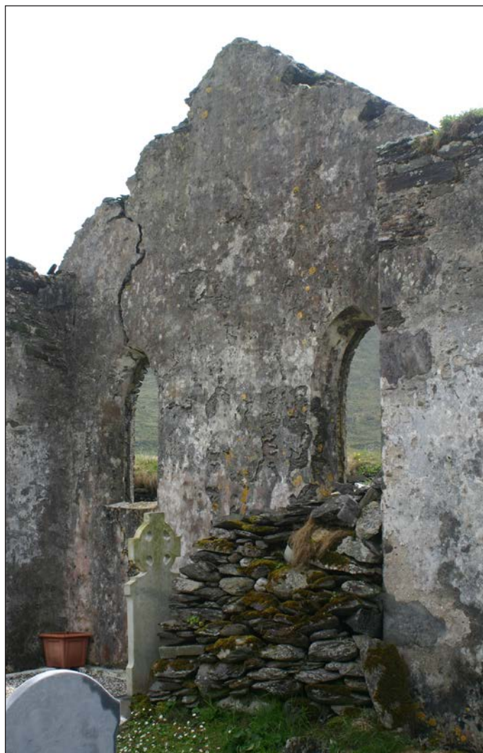
Plate 19: View of southern wall of 19th century church. Note large vertical crack extending upwards from easternmost window ope
