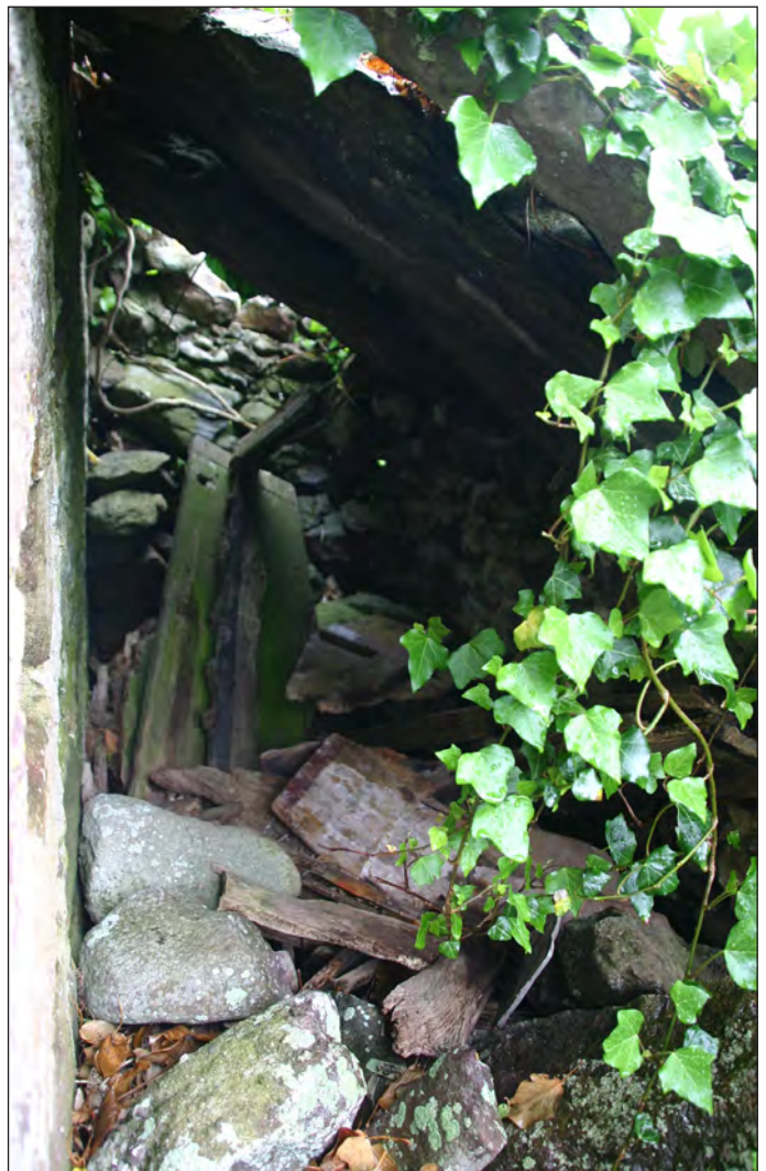
Plate 23: Close-up view of interior of narrow lean-to tomb immediately W of south doorway of church. Note partial collapse of tomb fabric and remains of wooden coffin(s)
