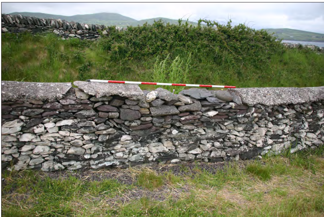
Plate 5: Close-up view of damaged and poorly repaired section of boundary wall at N
