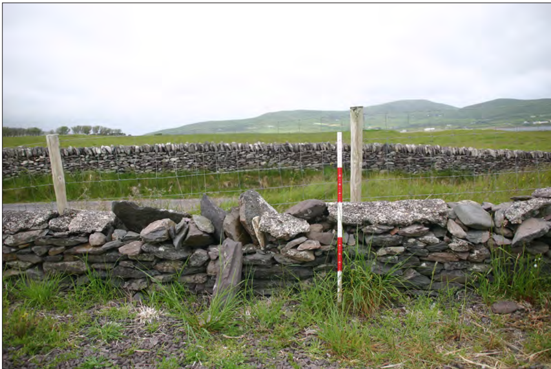
Plate 7: Close-up view of damaged and poorly repaired section of boundary wall at NE. Contrast damaged wall to drystone wall beyond
