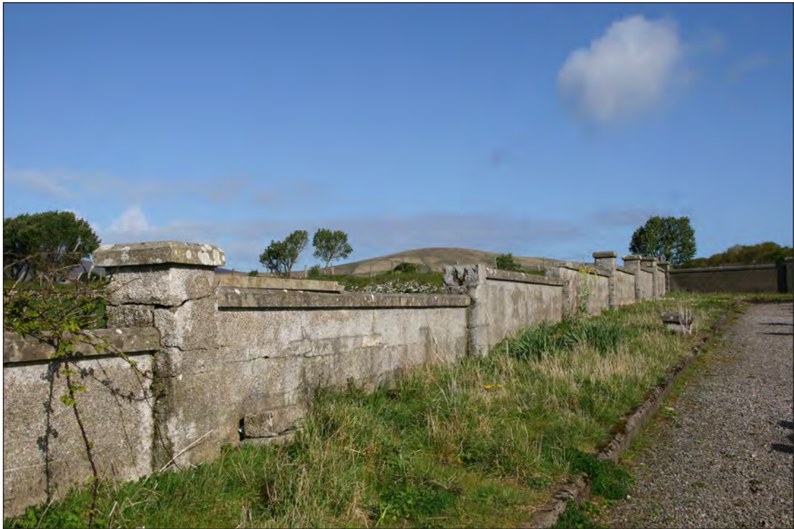
Plate 11: View of W boundary wall of new section of Ventry Graveyard. Note cracked piers and missing capping
