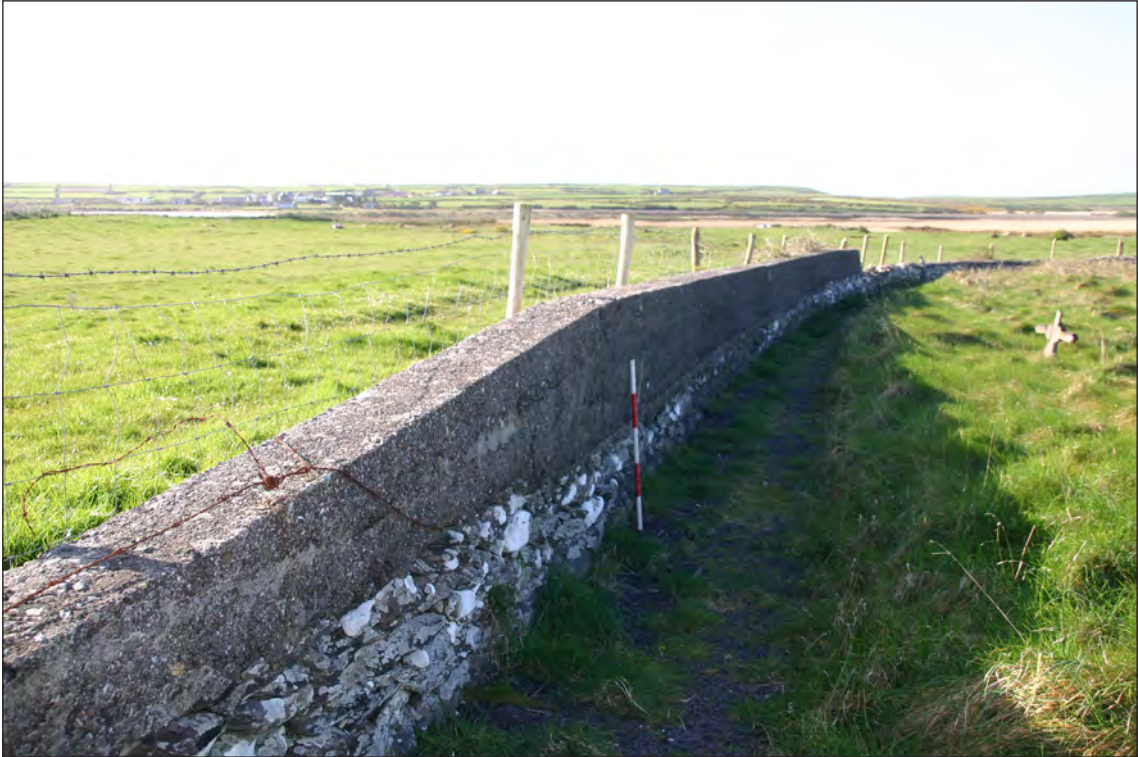
Plate 9: View of section of unsightly inappropriate mass-concrete walling on SSE limits of boundary wall
