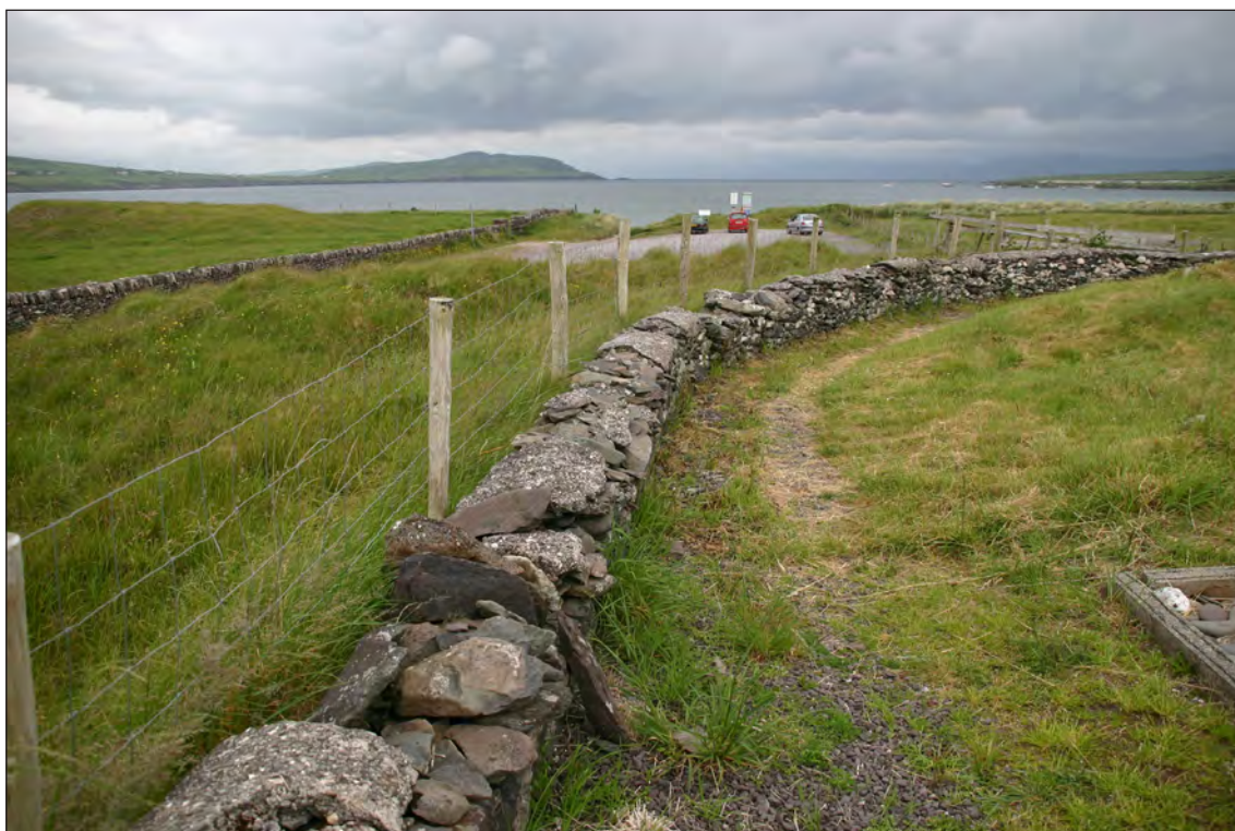
Plate 6: View of curving SE section of boundary wall at the medieval graveyard of Ventry. Note poor reduced condition and destroyed capping
