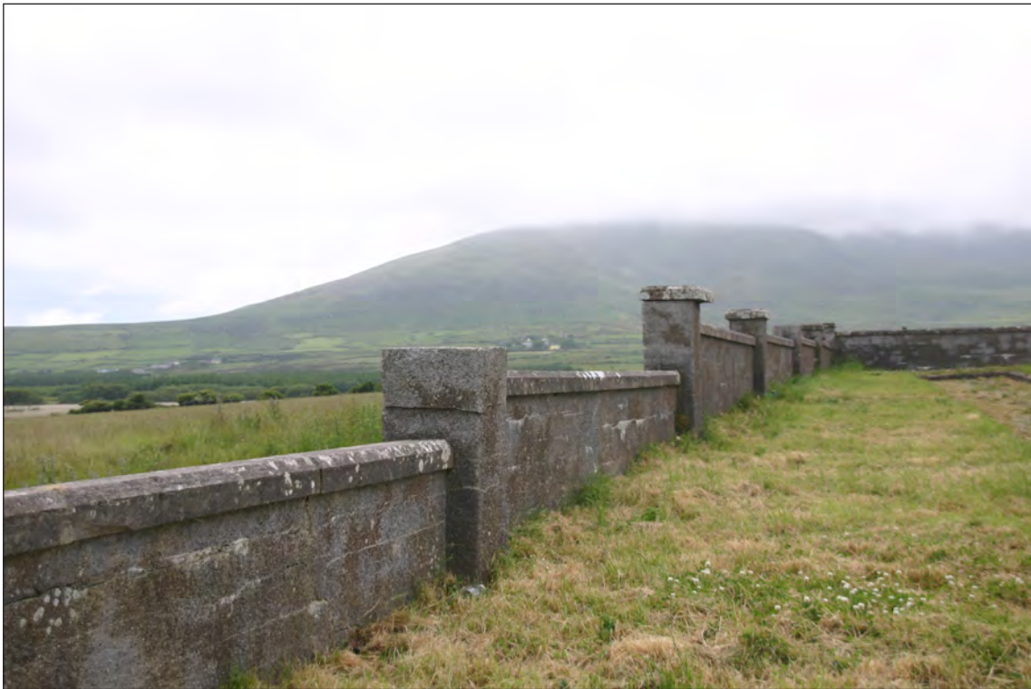
Plate 10: View of S boundary wall of new section of Ventry Graveyard. Note missing capping
