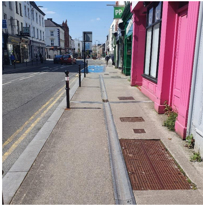
Figure 4.0 Accessible Spaces on Lower Castle Street
