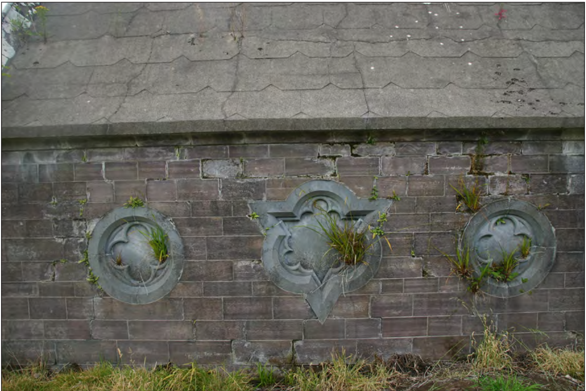
Plate 4: View of S elevation of 'Ventry' mausoleum. Note: growth in recessed limestone panels
