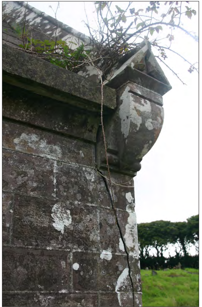
Plate 5: View of growth and severe crack on the gable shoulder and weather coping
