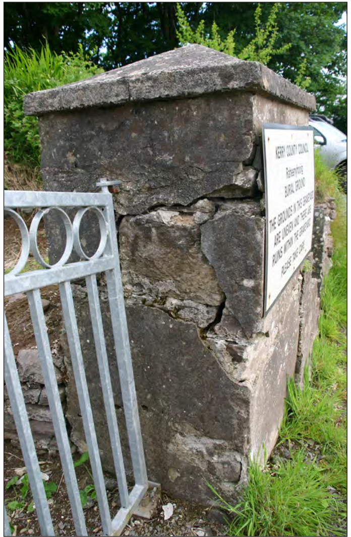
Plate 23: View of RH damaged entrance pier of Raheenyhooig Graveyard
