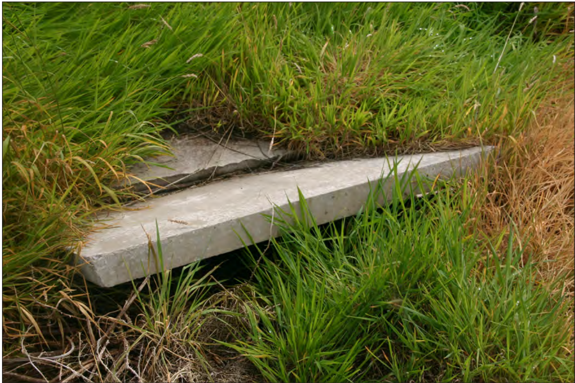
Plate 17: View of collapsing recently installed concrete lintels
