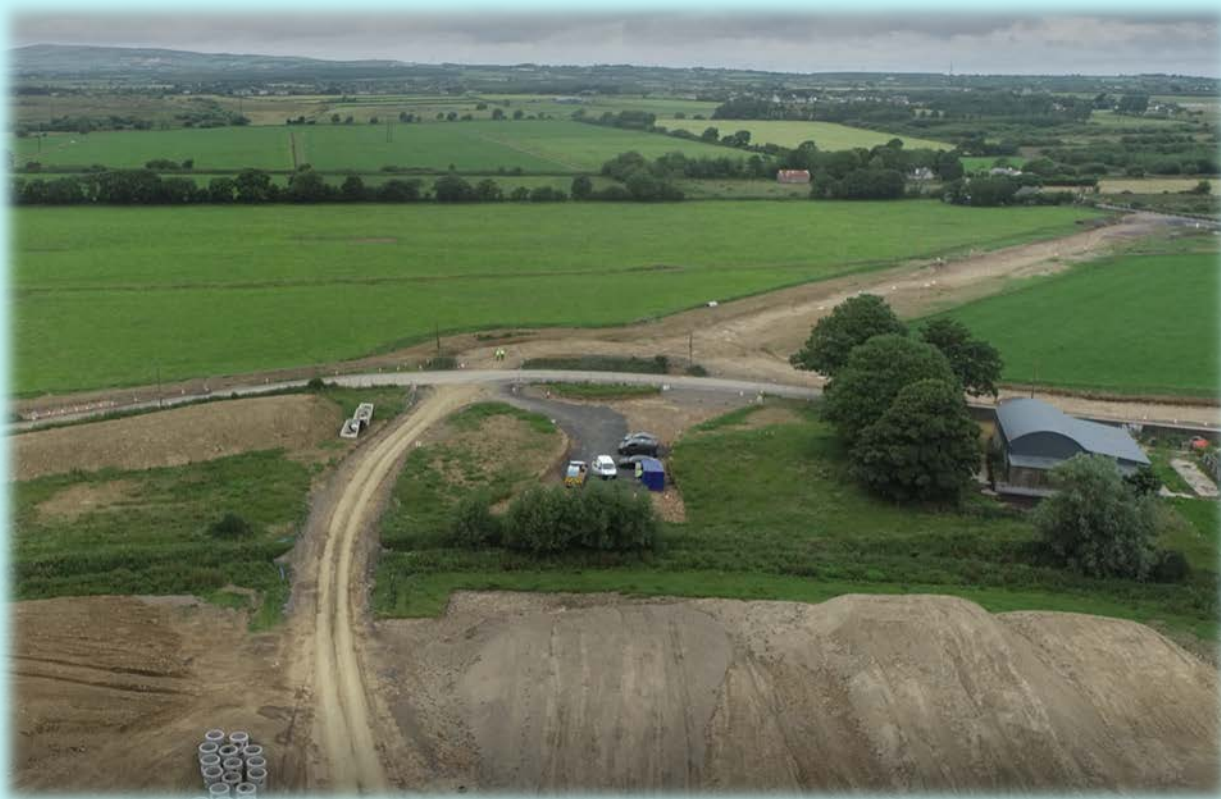
Figure 1-3 Greenville Road Roundabout to Forge Work
